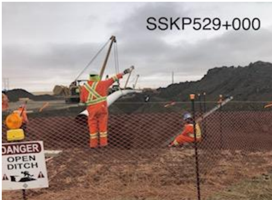
Lowering in a section near hotlines
