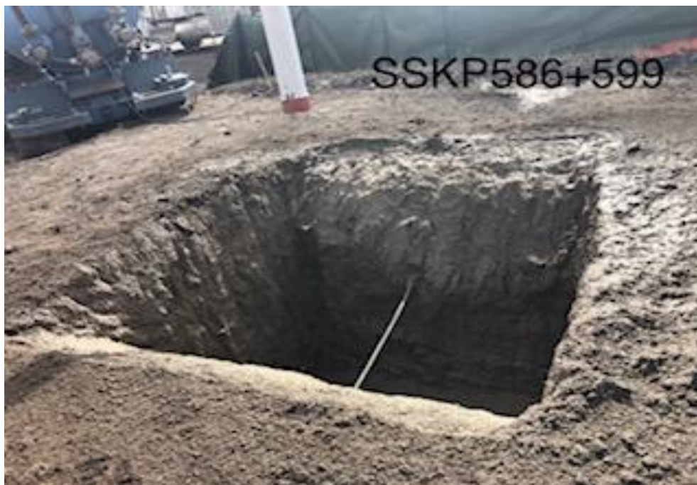
DAYLIGHTING SASK POWER CABLE
