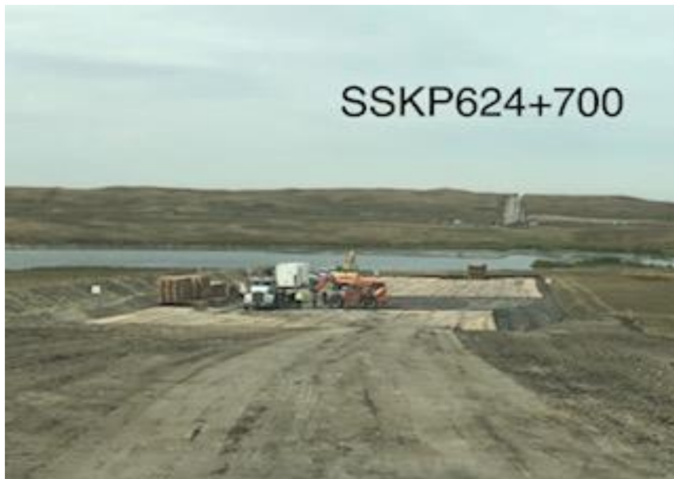
Ditch soil separation layer at Chapleau Lake
